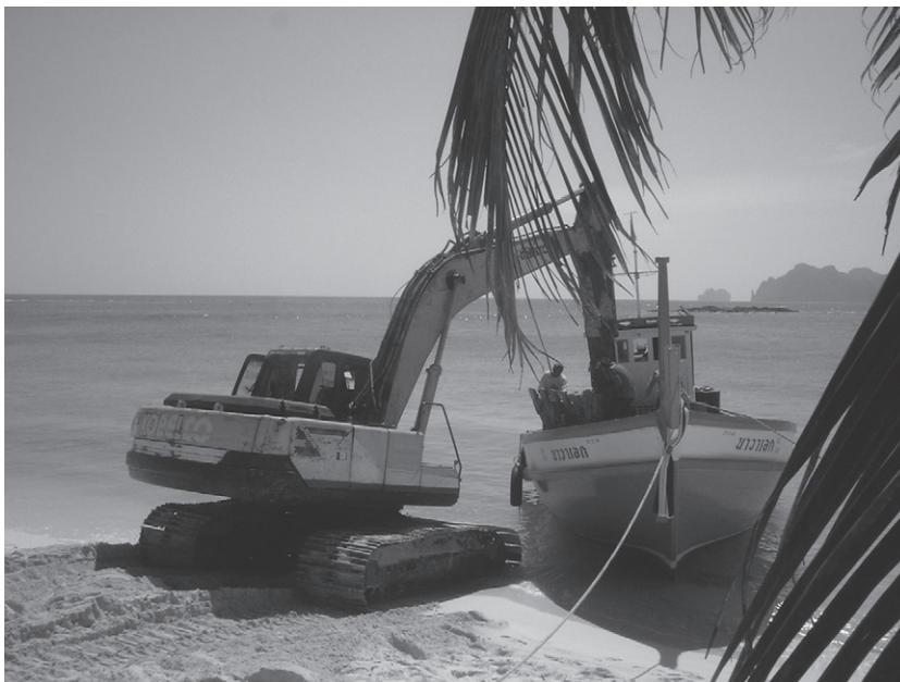
Plate 13 Unloading building materials for beach accommodation, Koh Phi Phi, Thailand.
