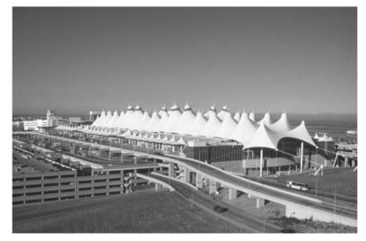
Denver International Airport exemplifies good planning for traveler convenience. The modern terminal building has separate dropoff levels for passengers arriving in private and commercial vehicles, close-in parking, and trains to shuttle passengers from the terminal to three concourses. *Photo courtesy* of Denver International Airport.
