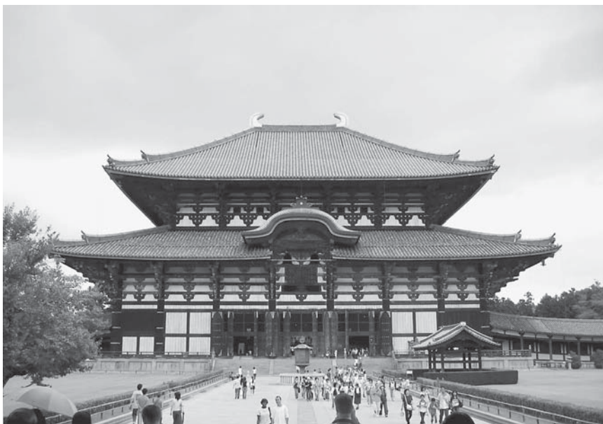
Figure 13.4 Todaiji Temple, Hall of the Great Buddha; founded 743, rebuilt in the 18th century, Nara, Japan. Courtesy of Shutterstock.
