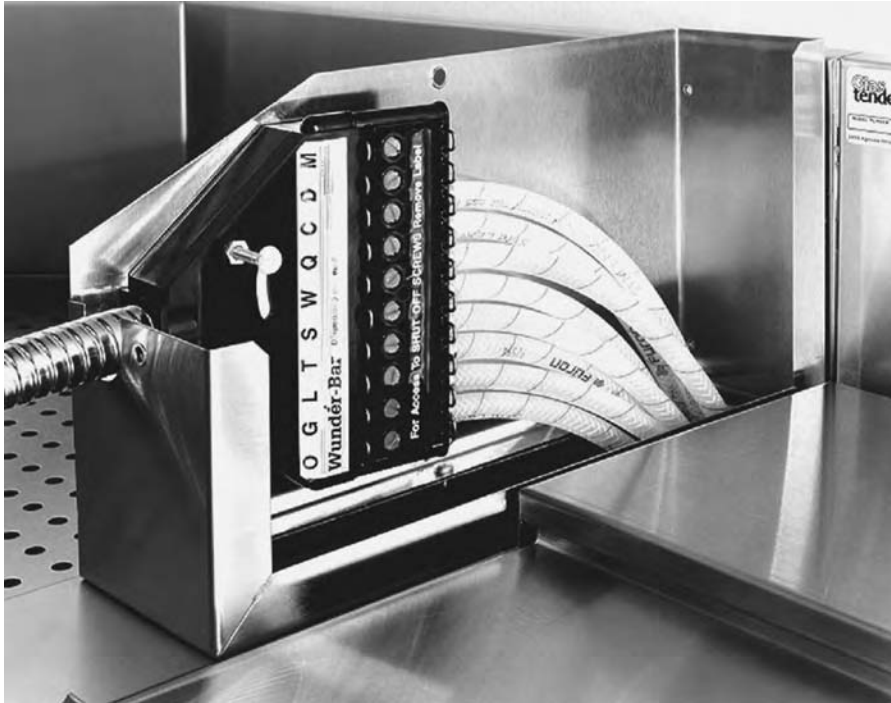
FIGURE 9.13 The series of hoses for a dispensing gun. Courtesy of Glastender, Inc., Saginaw, Michigan.
