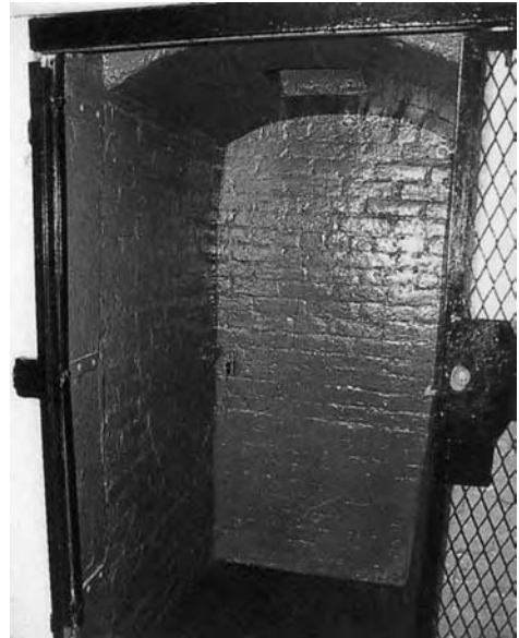
FIGURE 1.4 The trick door of New York’s ‘21’ Club, opened by pushing a metal bar into a tiny hole. Today the door still works and the area behind it is used as a wine cellar. Courtesy of the ‘21’ Club.
