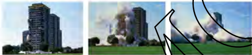
Figure 6.6 Explosives produce large quantities of high-pressure gas. When the gas expands, it does work by demolishing the building.
