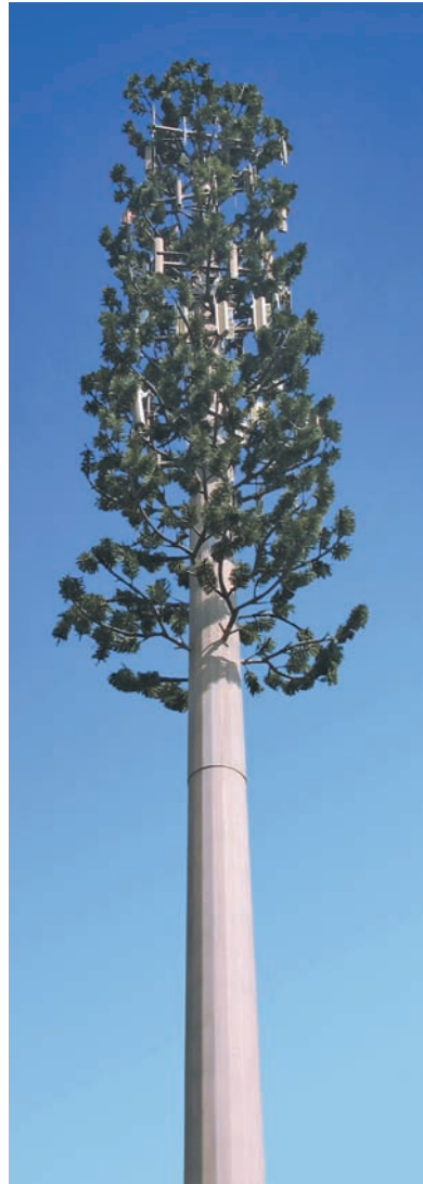
FIGURE 3-30 A cell tower disguised as a pine tree.
