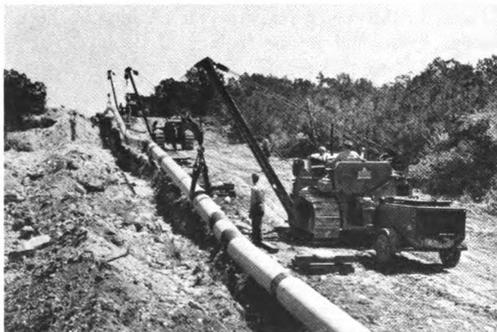
Fig. 6. Lowering-in a section of pipeline with three side-boom diesel tractors.
