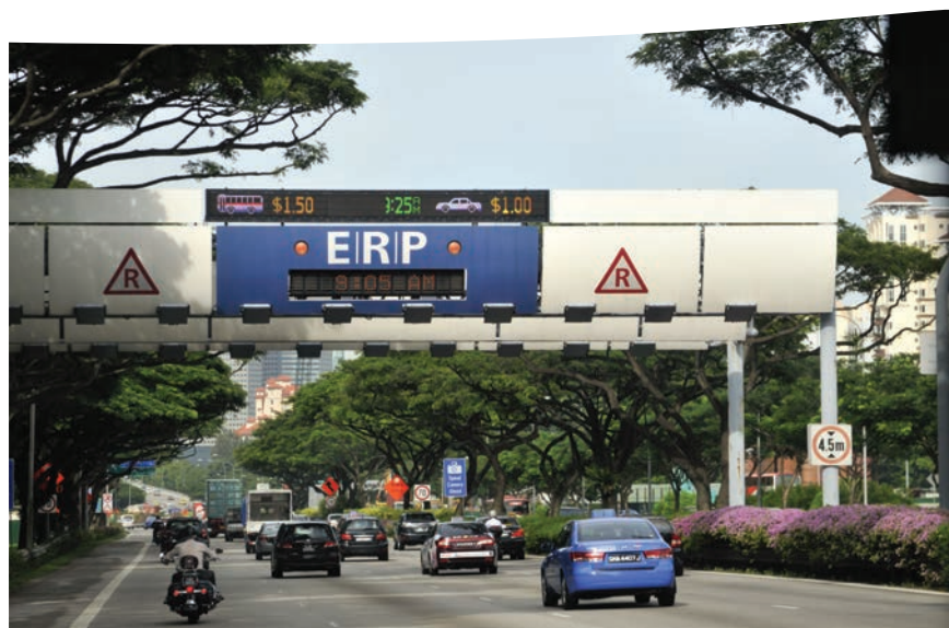
› Balancing private and public goods – In response to traffic congestion, Singapore has an electronic road pricing system where tolls are automatically deducted from prepaid cards placed in readers installed in all cars.
