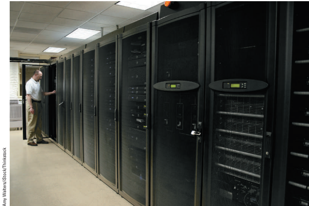
FIGURE 8-8 Rack-mounted blade servers
