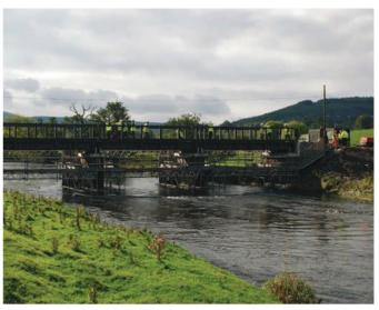
**Figure 21.34** The world's longest bridge made from recycled plastic. It was constructed in Peeblesshire in Scotland.
